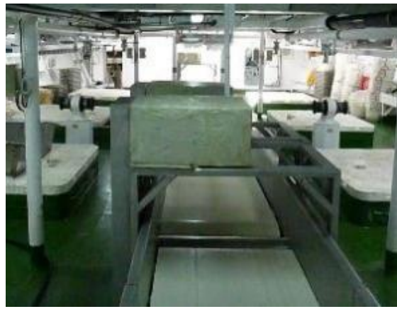
Figure 16: View from the forward viewing conveyor belt camera.
