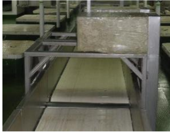
Figure 14: View from the midships aft facing conveyor belt camera.
